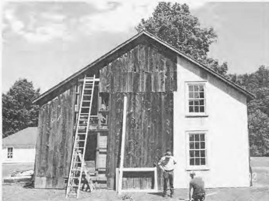
Museum Interpreter, Bill Brindle, and Mill Foreman, Robert Grassi, carefully measured and cut each board for the restoration of the south end of the Drying Shed. This photograph, taken on July 2, 2004, shows original boards in the middle and on the left, and new boards on the right. They are replacing the boards where the ladder is standing.
